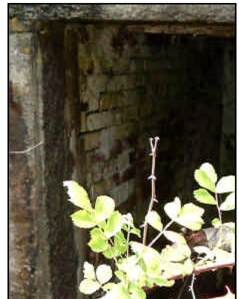
Poor house tomb that became an office.
